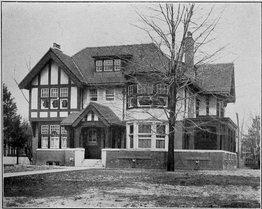
Residence at Detroit, Mich. Mildner and Eisen, Architects, Detroit
