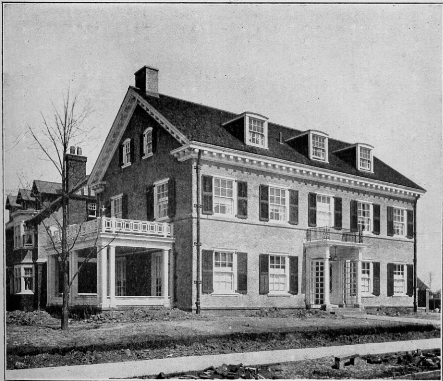
House at Detroit, Mich. Stratton & Baldwin Architects, Detroit M. R. Burrowes, Associate
