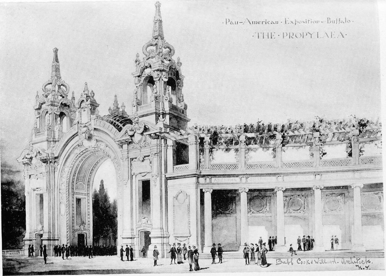
THE PROPYLÆA, PAN-AMERICAN EXPOSITION, BUFFALO, N. Y. BABB, COOK & WILLARD, Architects, New York.
