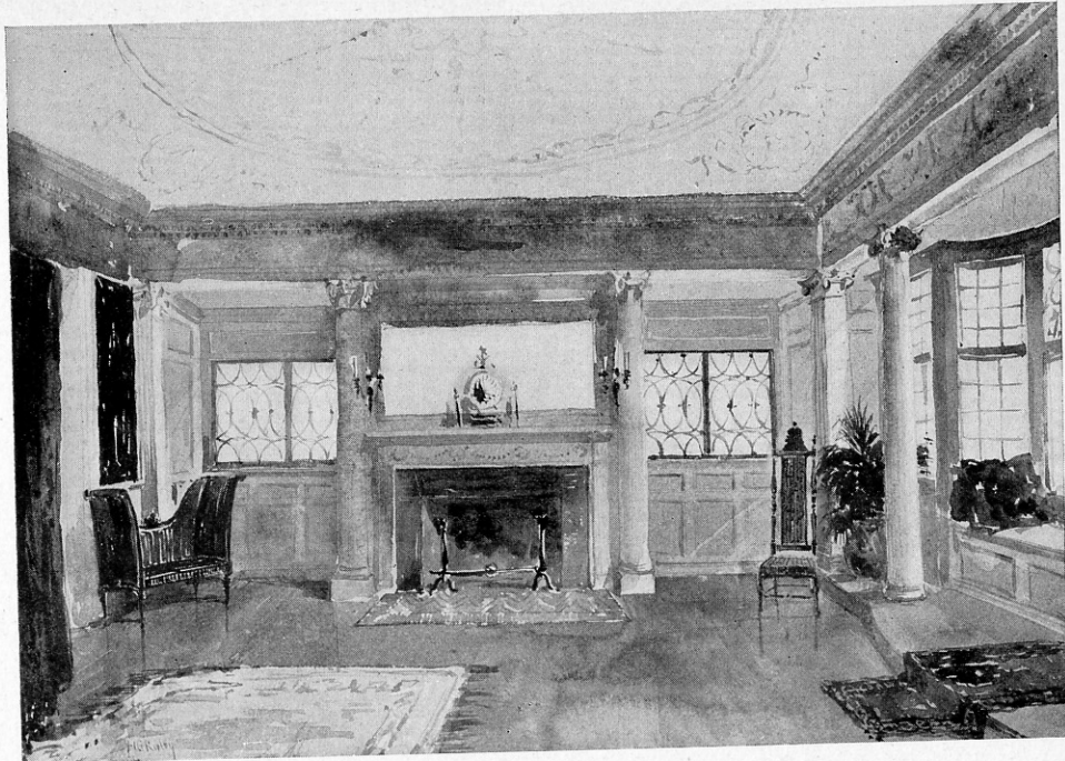
RECEPTION HALL, RESIDENCE OF MR. W A BUTLER, DETROIT, MICH. CHAPMAN & FRAZER, Architects, Boston.
