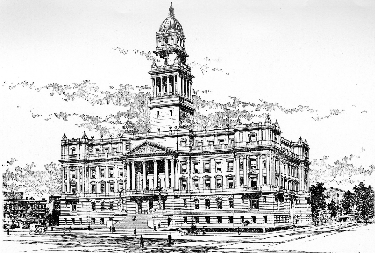
NEW WAYNE COUNTY BUILDING, DETROIT, MICH. JOHN SCOTT & Co., Architects, Detroit.
