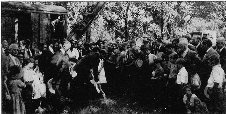
TURNING THE FIRST SOD
